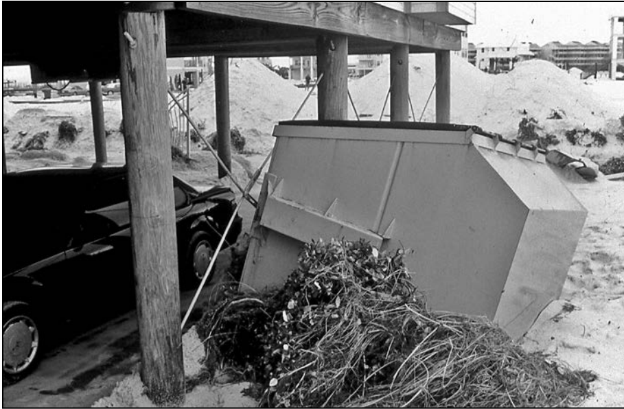
Figure 14: Floating debris trapped by metal rod cross bracing
