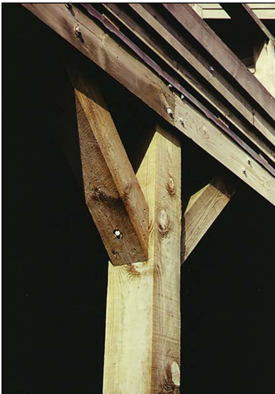
Figure 15: Knee bracing
