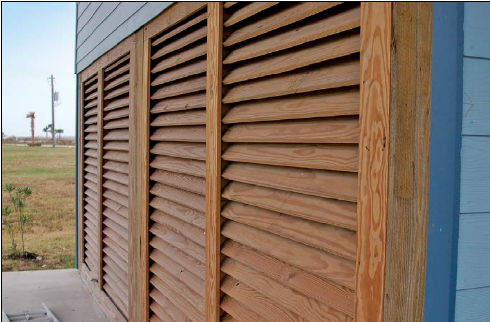
Figure 5: Compliant, fixed, wood louvers installed between pilings
