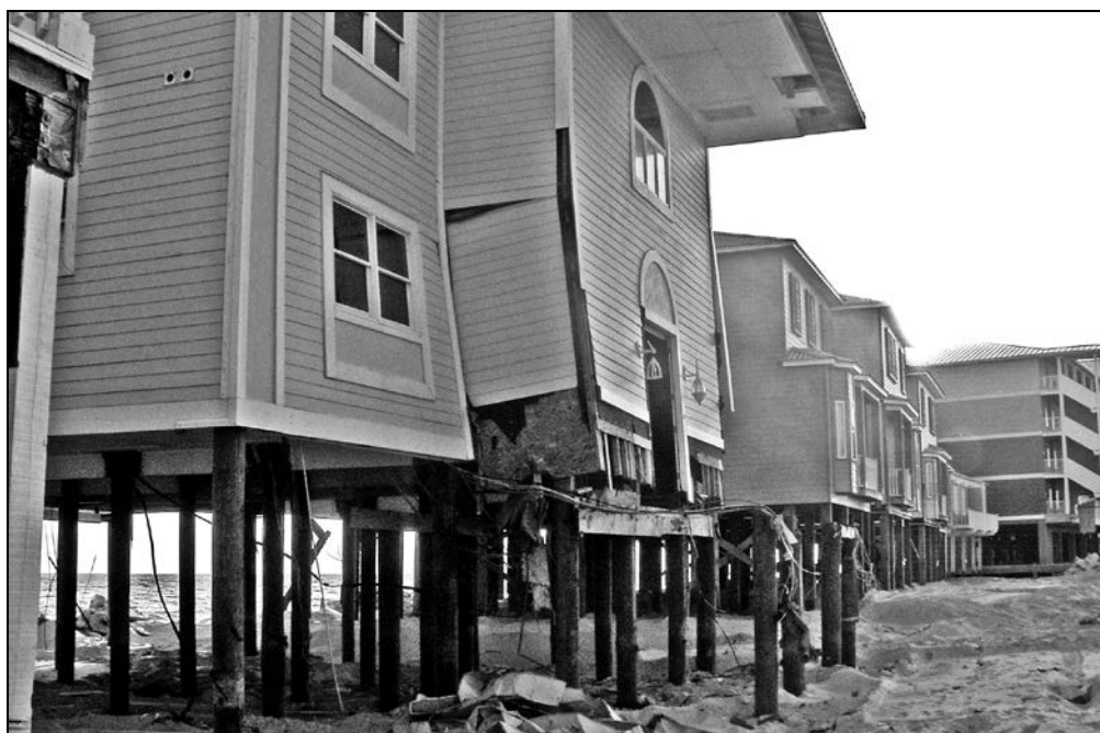
Figure 1: Damage to an elevated building as a result of stairs that did not break away cleanly
