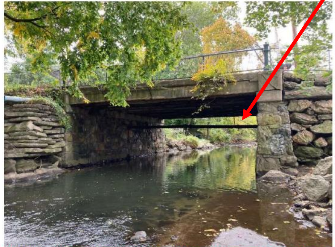
Figure 4-13: Looking upstream at Tompkins Avenue bridge. Passage across the bridge has been closed off due to structural concerns. A utility line is seen suspended underneath the bridge deck at the inlet.
